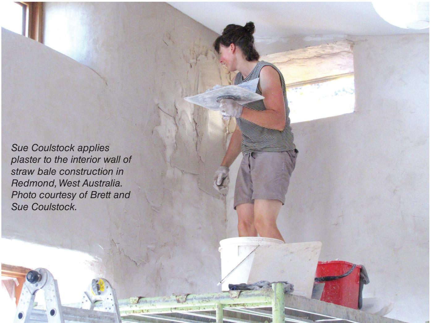
*Sue Coulstock applies plaster to the interior wall of straw bale construction in Redmond, West Australia. Photo courtesy of Brett and Sue Coulstock.*
